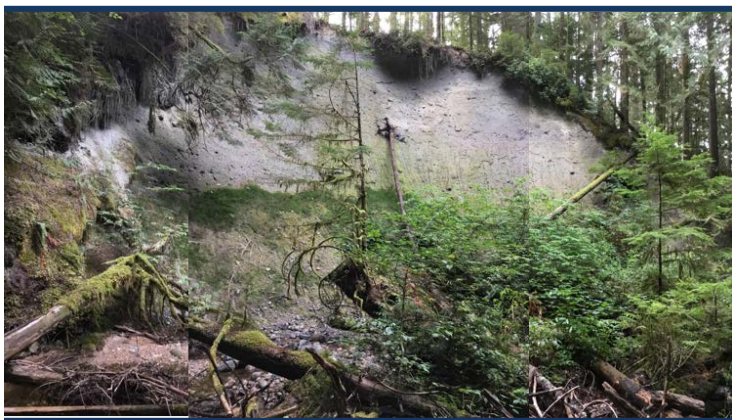
Picture 1. The retrogressive slump adjacent to Wilson Creek. Note the revegetation of the toe of the slump.
