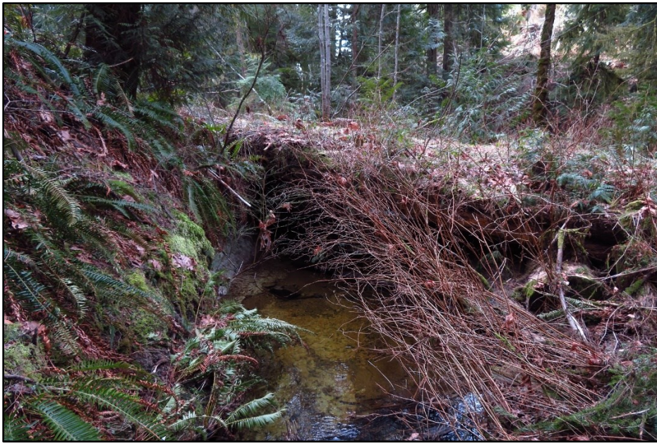
Photo 9: Collapsing log stringer private land bridge downstream of Leaning Tree Road
