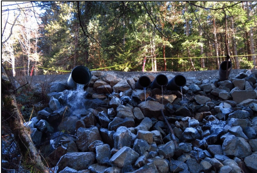
Photo 3: New metal and plastic pipe culverts
