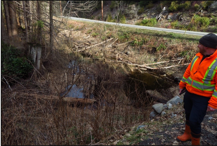
Photo 8: Strandline shows extent of ponding during flood upstream of Belair Road
