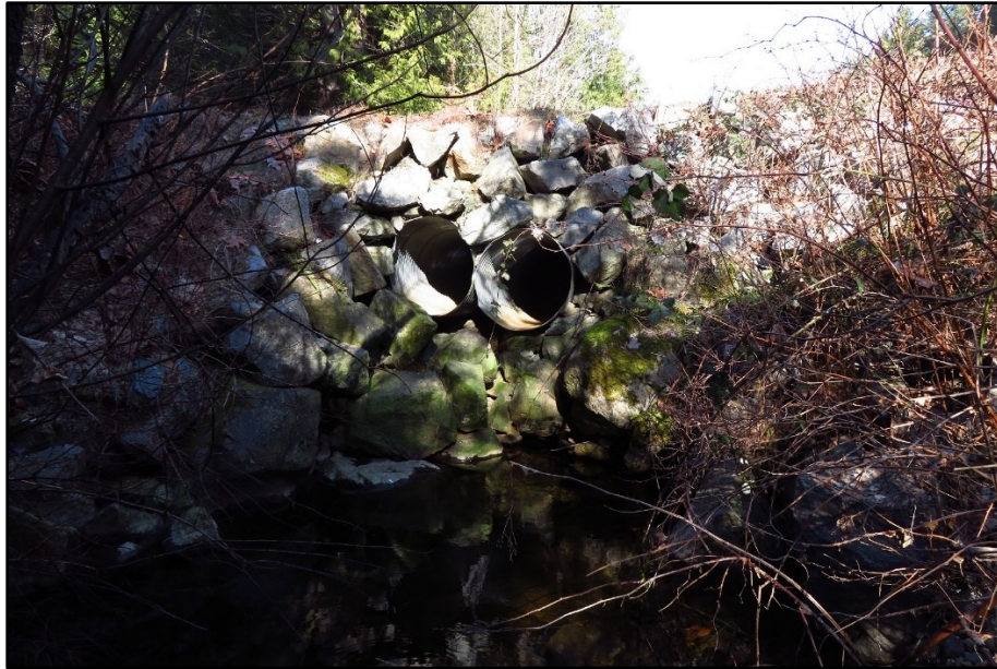
Photo 6: Double culverts at Leaning Tree Road stream crossing
