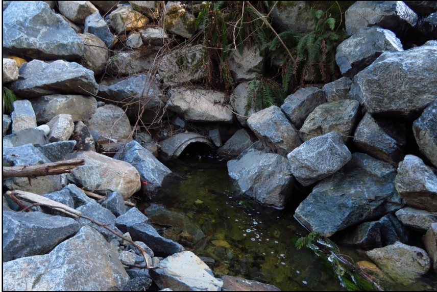
Photo 2: Concrete culvert at base of Redrooffs Road fill
