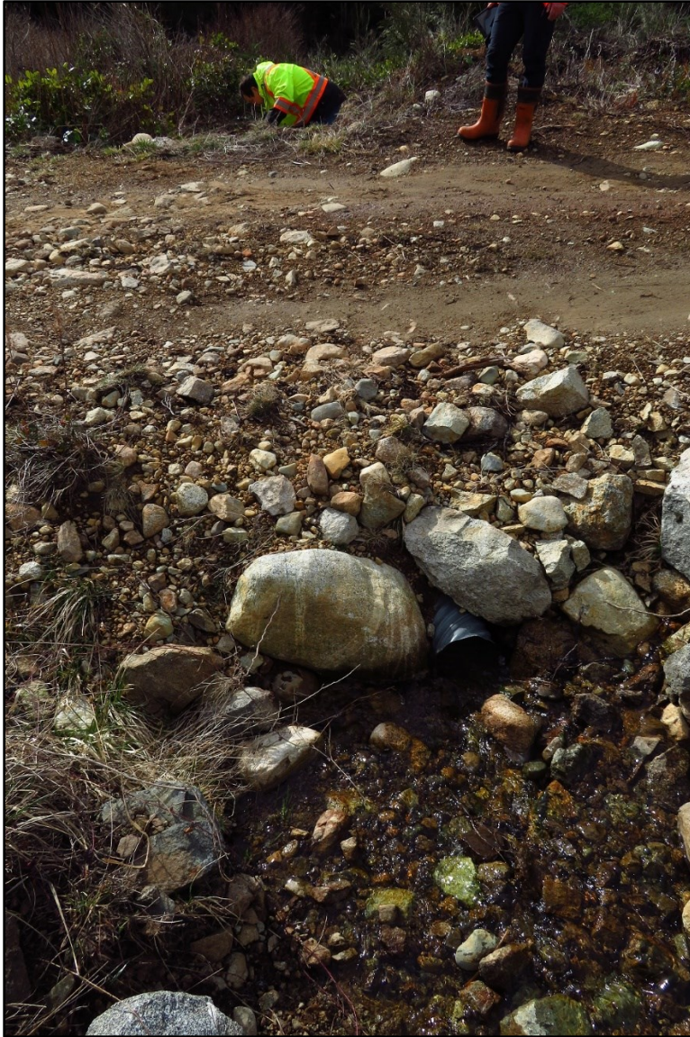
Photo 16: Tiny culvert under BC Hydro access road
